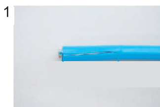
Expose inner vinyl sheath.
